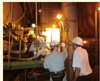
Installing the heat-resistant camera inside the boiler (Photo Credit: Security Japan Co. Ltd.)
